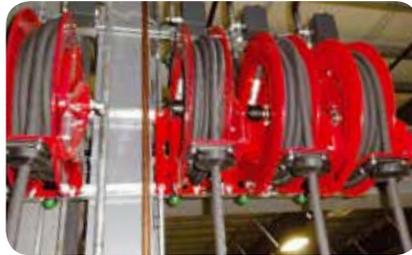
*Hose reels are locked out by solenoids. Each dispense request opens up a solenoid valve, activating a green ready light, indicating the dispense is ready to proceed.*
