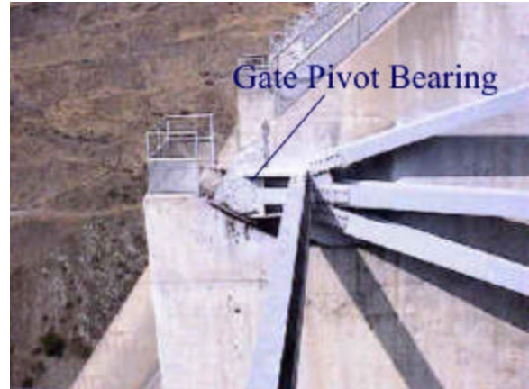
View of the Gate Pivot Bearing. The Divider Valve is located at the base of the bearing.
