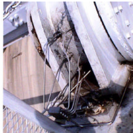
Close up view of the Divider Valve with lines going into eight grease points.
